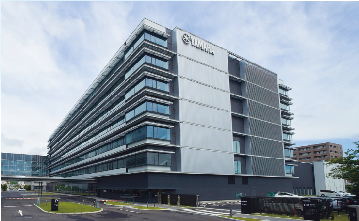
Yamaha Corporation Headquarters Building No.21 Air Conditioning System (Hamamatsu City, Shizuoka Prefecture)
