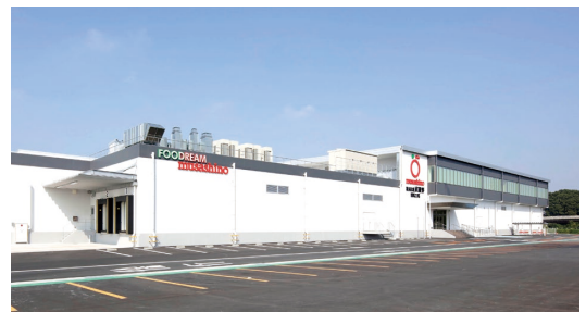
Musashino Co., Ltd. Gunma Factory Air Conditioning and Sanitation Systems and utility facilities (Takasaki City, Gunma Prefecture)
