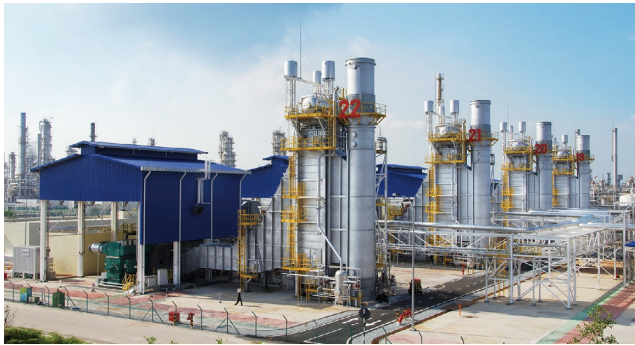
Petronas Penapisan (Melaka) Sdn Bhd Cogeneration Plant Plant Facilities (Malaysia)
