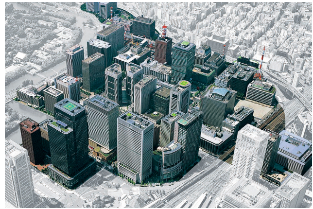
Otemachi District, Marunouchi 1-chome District DHC District Heating and Cooling System (Chiyoda-ku, Tokyo)
