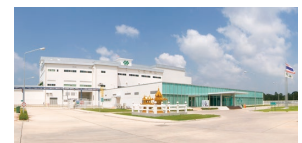
THAI KYOWA BIOTECHNOLOGIES CO., LTD. Plant facilities/civil engineering and construction (Thailand)
