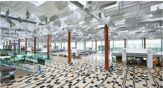
Changi International Airport Terminal 3 "Courtesy of Civil Aviation Authority of Singapore" Air Conditioning and Mechanical Ventilation System (Singapore)
