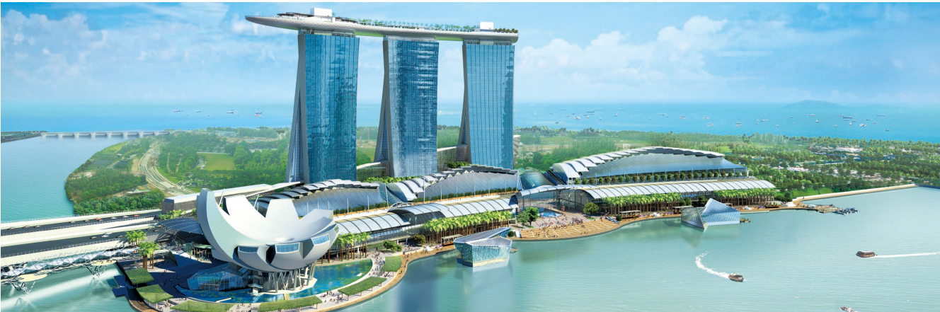
Marina Bay Sands Integrated Resort Air Conditioning and Mechanical Ventilation System (Singapore)
