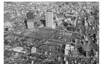
Shinjuku Fukutoshin District District Heating and Cooling System
