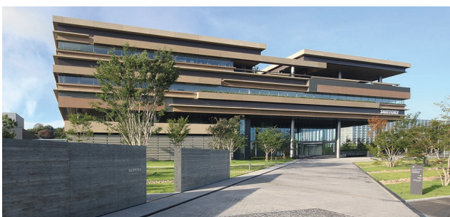
SUNTORY WORLD RESEARCH CENTER Sanitation System (Soraku-gun, Kyoto)
