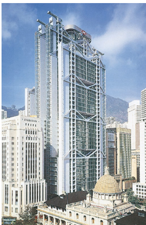
The Hong Kong and Shanghai Banking Corporation Limited, HSBC Main Building Air conditioning, sanitation and electric system (Hong Kong)
