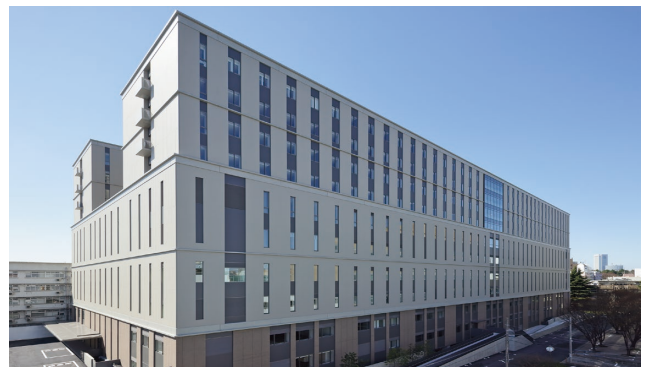
Keio University Hospital Bldg. 1 Air Conditioning System (Shinjuku-ku, Tokyo)
