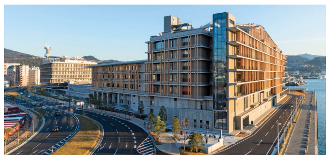
Nagasaki Prefecture office administrative building Air Conditioning System (Nagasaki City, Nagasaki Prefecture)
