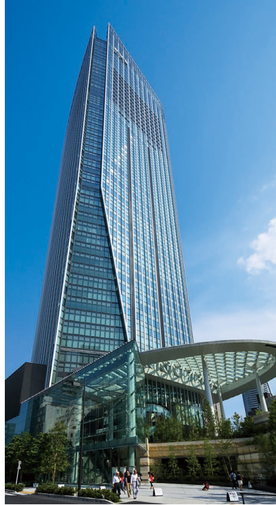
Toranomon Hills Air Conditioning System (Minato-ku, Tokyo)
