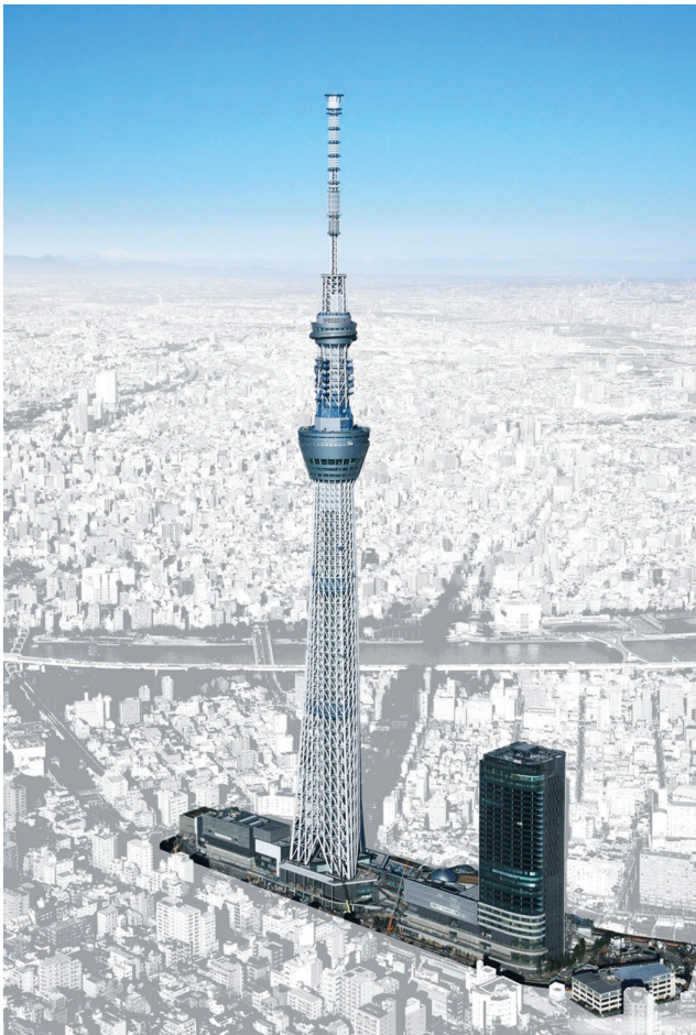
Tokyo Sky Tree® District DHC District Heating and Cooling System (Sumida-ku, Tokyo)
