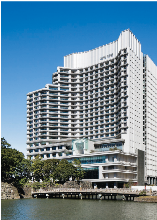
Palace Hotel Tokyo - Palace Building Air Conditioning System (Chiyoda-ku, Tokyo)
