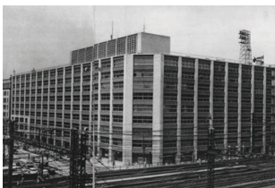
Shin-Otemachi Building Air conditioning system
