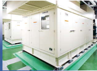
Gas engine CGS
