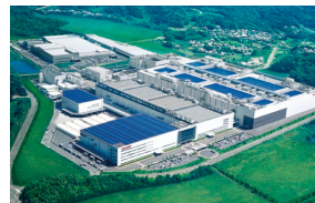
Sharp Corporation Kameyama Factory Air conditioning System
