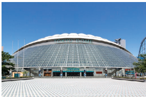
Tokyo Dome Air conditioning System
