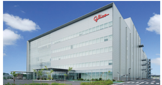
Kanto Glico Co., Ltd. Kitamoto Factory Air Conditioning and Sanitation Systems (Kitamoto City, Saitama Prefecture)
