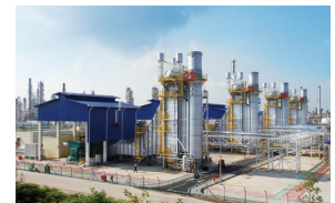
Petronas Penapisan (Melaka) Sdn Bhd Cogeneration Plant Plant facilities (Malaysia)
