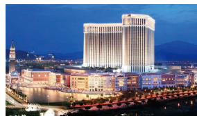
The Venetian Macao Resort Air conditioning/district heating and cooling system (Macau)
