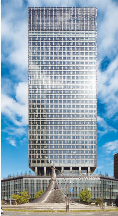
Dai Nagoya Building Air Conditioning System (Nagoya City, Aichi Prefecture)
