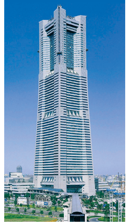
THE LANDMARK TOWER YOKOHAMA Air Conditioning System (Yokohama City, Kanagawa Prefecture)
