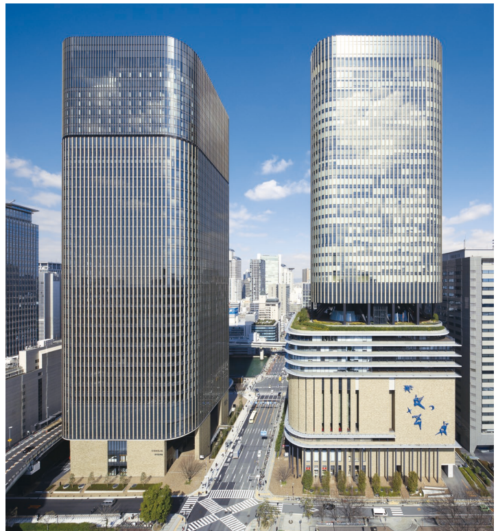
FESTIVAL CITY Air Conditioning/District Heating and Cooling System (Osaka City, Osaka)
