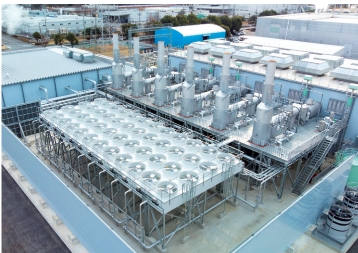
Auxiliary Equipment Area (Around the Exhaust Gas Boilers/Radiators)
