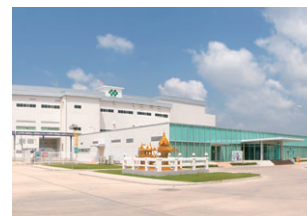
THAI KYOWA BIOTECHNOLOGIES CO., LTD. Plant facilities/civil engineering and construction (Thailand)
