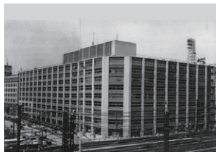
Shin-Otemachi Building Air conditioning system
