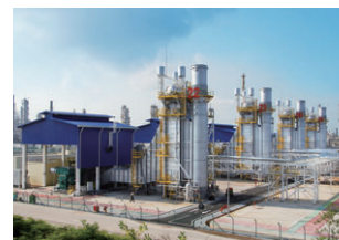
Petronas Penapisan (Melaka) Sdn Bhd Cogeneration Plant Plant facilities (Malaysia)
