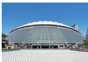
Tokyo Dome Air conditioning System
