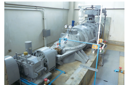
Pump After Servicing
