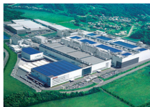
Sharp Corporation Kameyama Factory Air conditioning System
