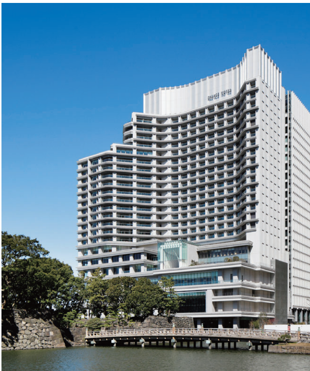
Palace Hotel Tokyo - Palace Building (Chiyoda-ku, Tokyo)
