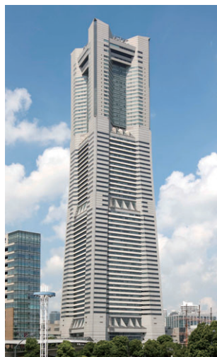
THE LANDMARK TOWER YOKOHAMA Air conditioning System
