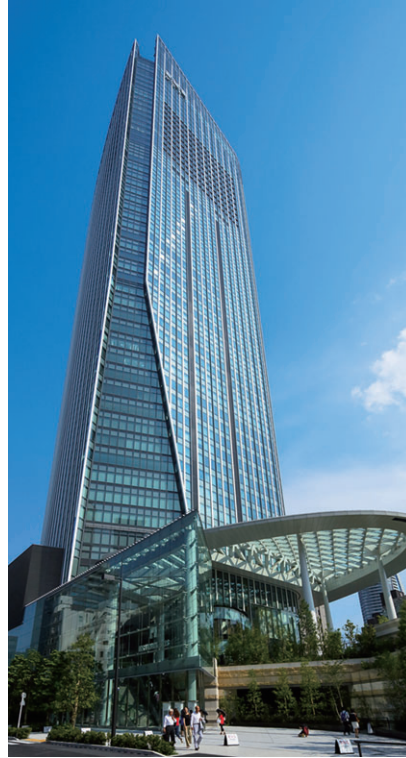
Toranomon Hills Mori Tower (Minato-ku, Tokyo)
