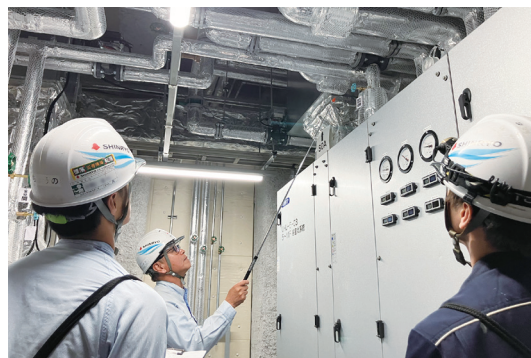
Confirming Status of Piping and Valve Constructions
