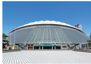
Tokyo Dome Air conditioning System
