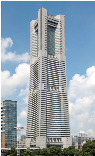
THE LANDMARK TOWER YOKOHAMA Air conditioning System
