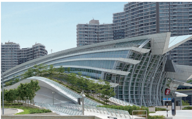
Hong Kong West Kowloon Station, Guangzhou-Shenzhen-Hong Kong Express Rail Link (Hong Kong)
