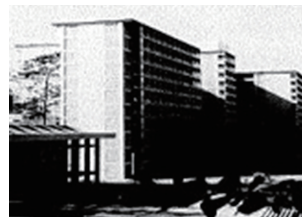
Cho-Ray Hospital Air conditioning and sanitation Systems (Vietnam)
