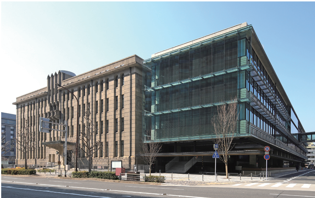
Exterior of the Northern Government Office
