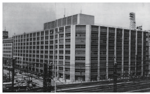
Shin-Otemachi Building Air conditioning System
