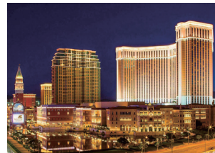
The Venetian Macao Resort Air conditioning/District Heating and Cooling System (Macau)
