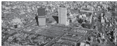
Shinjuku Fukutoshin District District Heating and Cooling System
