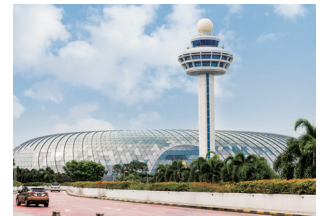
Jewel Changi Airport Air conditioning and Mechanical ventilation Systems (Singapore)
