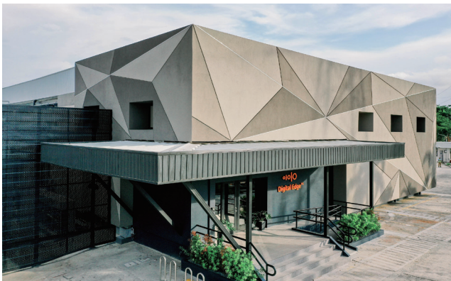
NARRA1 Data Center (Philippines)
