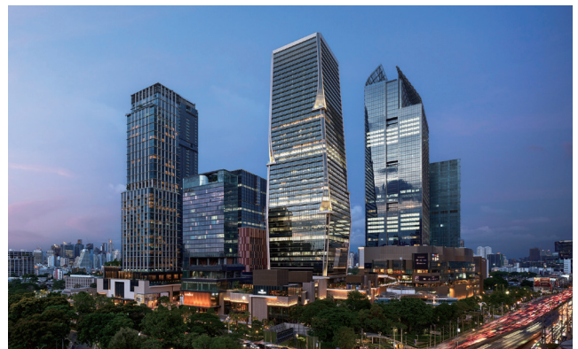
District Cooling Plant for One Bangkok (Thailand)
