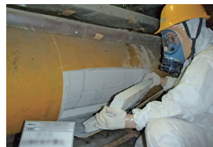
Removal of Piping Insulation Containing Asbestos
