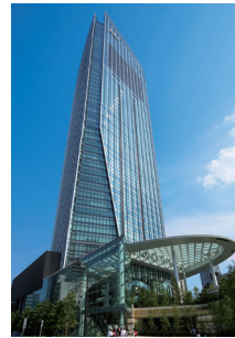
Toranomon Hills Mori Tower Air conditioning System
