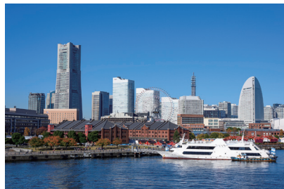
District heating and cooling systems
