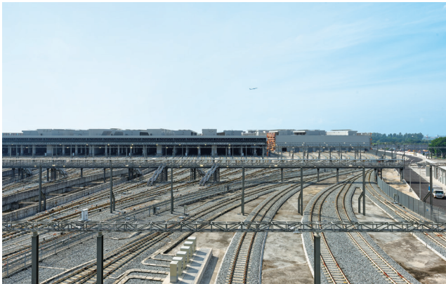
Exterior of the Train Depot
