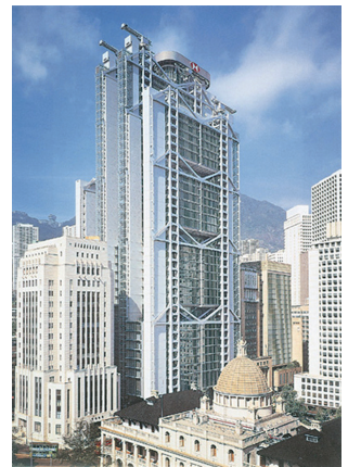
The Hong Kong and Shanghai Banking Corporation Limited, HSBC Main Building Air-conditioning, Sanitation, and Electric Systems (Hong Kong)
