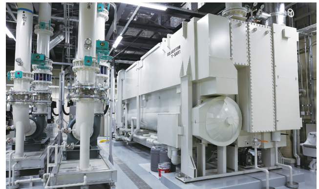
Steam absorption chiller
