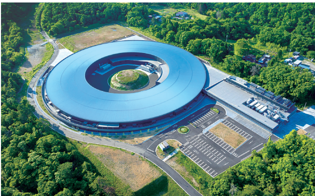
3GeV Synchrotron Radiation Facility "NanoTerasu" (Sendai City, Miyagi)
