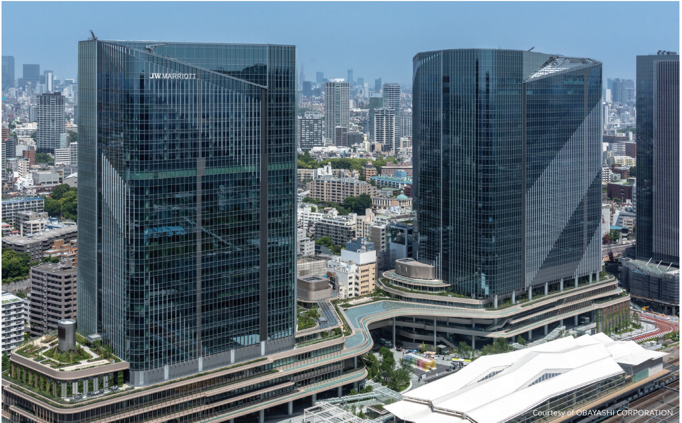
Building exterior (left side)
