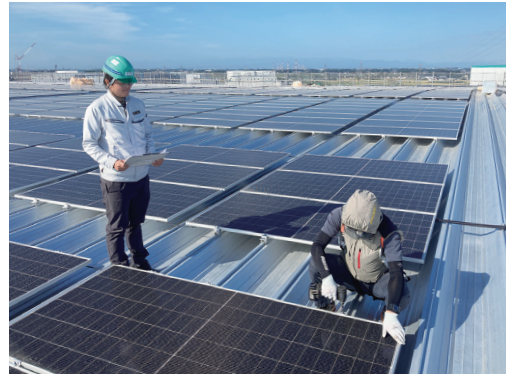
Confirming the installation of solar photovoltaic panels
