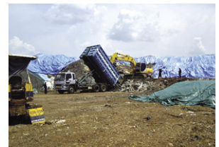
Landfilling asbestos slate tiles at a waste disposal site
