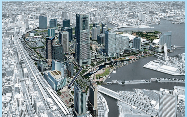
Minato Mirai 21 Central District DHC (Yokohama City, Kanagawa Prefecture)
