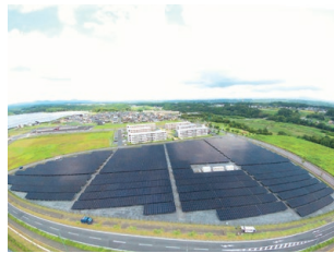
Ideal place for photovoltaic power generation systems
