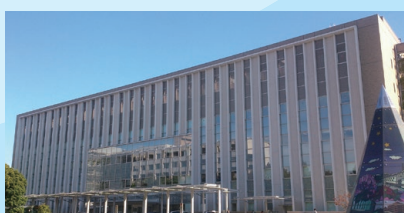
Hiroshima University Hospital Clinic Building (Hiroshima City, Hiroshima Prefecture)
