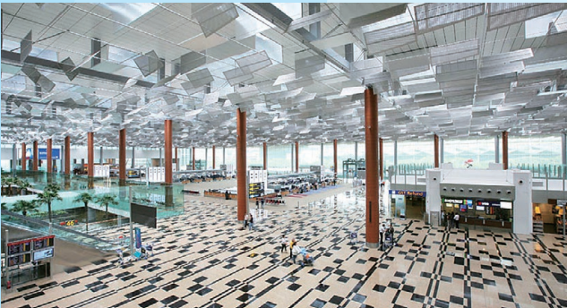
Changi International Airport Terminal 3 (Singapore) "Courtesy of Civil Aviation Authority of Singapore"
