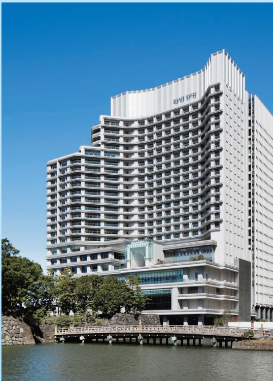
Palace Hotel Tokyo・Palace Building (Chiyoda-ku, Tokyo)
