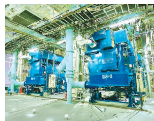
Point cloud data measured using a 3D laser scanner
