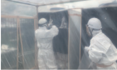
Removal Operations for Products that Contain RCF
