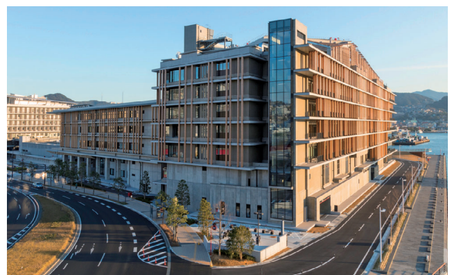
Nagasaki Prefecture office administrative building (Nagasaki City, Nagasaki Prefecture)
