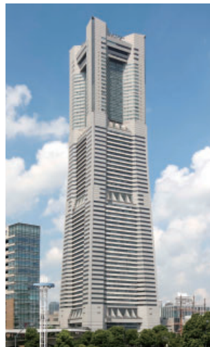
THE LANDMARK TOWER YOKOHAMA Air conditioning System
