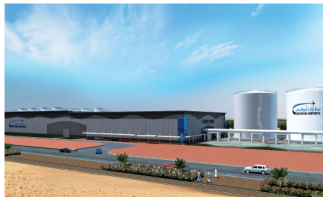
District Cooling Plant for the New Abu Dhabi International Airport Terminal (United Arab Emirates)
