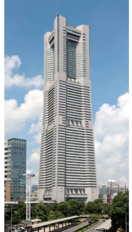
THE LANDMARK TOWER YOKOHAMA (Yokohama City, Kanagawa Prefecture) Air Conditioning System
