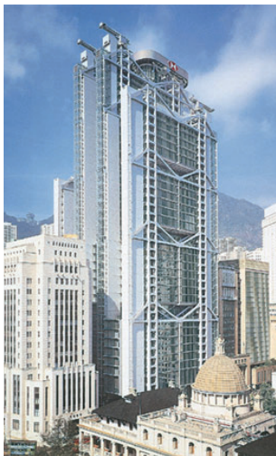
The Hong Kong and Shanghai Banking Corporation Limited, HSBC Main Building Air conditioning, sanitation and electric system (Hong Kong)
