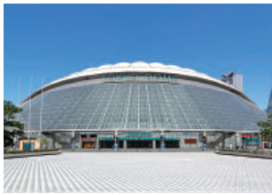
Tokyo Dome Air conditioning System
