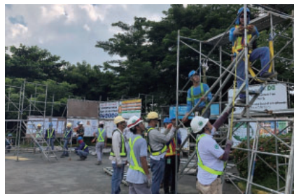
Assembly Drill for Construction Scaffolding
