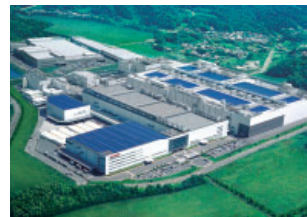
Sharp Corporation Kameyama Factory Air conditioning System
