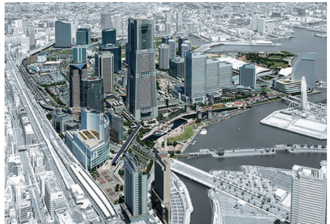
Minato Mirai 21 Central District DHC (Yokohama City, Kanagawa Prefecture)
