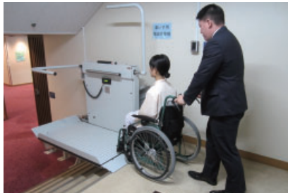
Stair Elevator for Wheelchair Use
