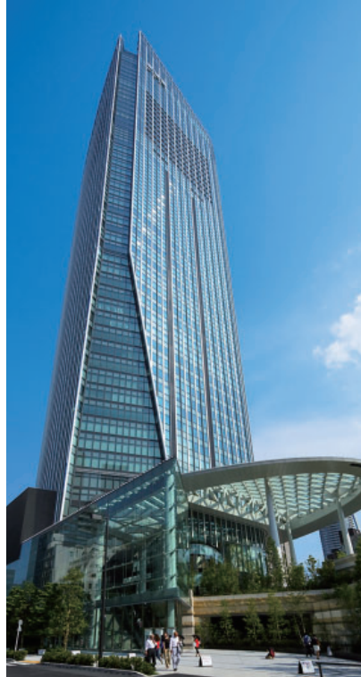
Toranomon Hills (Minato-ku, Tokyo) Air Conditioning System
