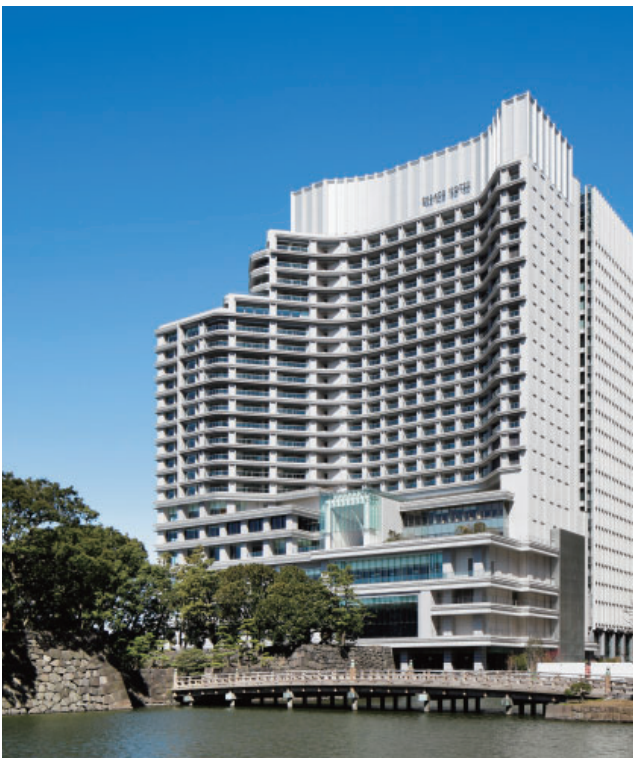
Palace Hotel Tokyo - Palace Building (Chiyoda-ku, Tokyo) Air Conditioning System
