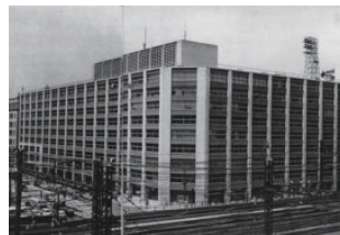
Shin-Otemachi Building Air conditioning system
