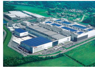
Sharp Corporation Kameyama Factory Air conditioning System
