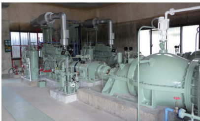
Shimo Ogawa Drainage Pump Station After Restoration
