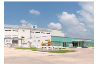
THAI KYOWA BIOTECHNOLOGIES CO., LTD. Plant facilities/civil engineering and construction (Thailand)
