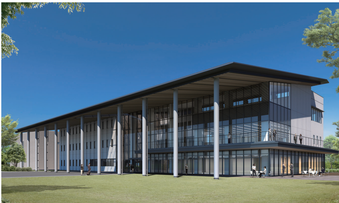
Main Building Mock Up of the New Research and Development Center
