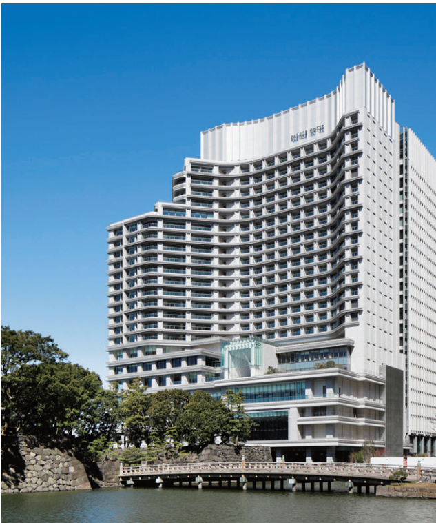
Palace Hotel Tokyo · Palace Building (Chiyoda-ku, Tokyo)
