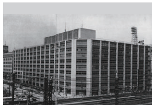
Shin-Otemachi Building Air conditioning system
