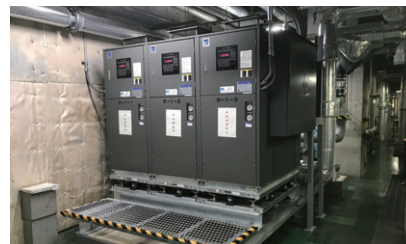
High-efficiency Equipment Upgrade Handled by Shinryo Technical Service
