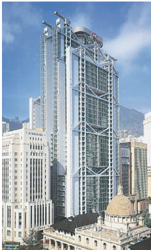
The Hong Kong and Shanghai Banking Corporation Limited, HSBC Main Building Air conditioning, sanitation and electric system (Hong Kong)
