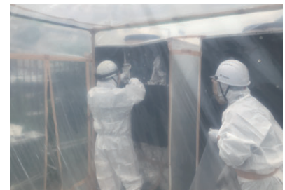
Removal Operations for Products that Contain RCF
