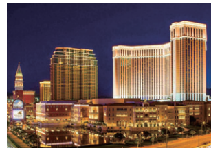
The Venetian Macao Resort Air conditioning/District Heating and Cooling system (Macao)
