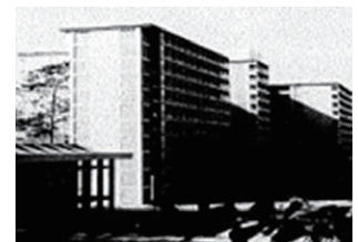
Cho-Ray Hospital Air conditioning and sanitation systems (Vietnam)
