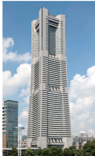
THE LANDMARK TOWER YOKOHAMA Air conditioning System
