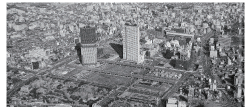
Shinjuku Fukutoshin District District Heating and Cooling System
