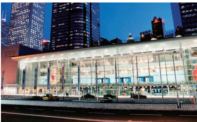
Hong Kong MTRC Airport Express Hong Kong Station (Hong Kong)
