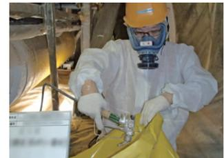
Spray and Disposal of an Agent to Prevent the Scattering of Asbestos
