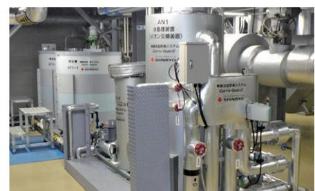
External View of the Corro-Guard® Non-chemical Corrosion Prevention System
