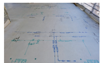
Floor after drawing completed
