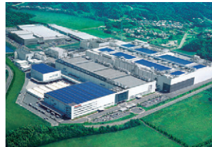
Sharp Corporation Kameyama Factory Air conditioning System
