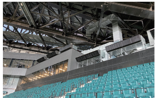
Air conditioning starts
