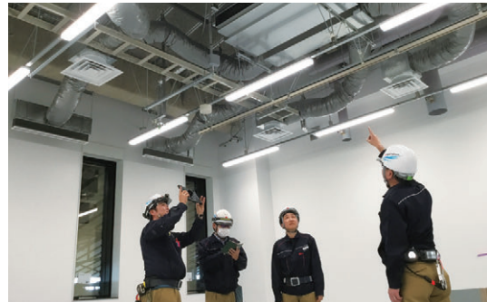
Confirming Construction Status Through Quality Patrols
