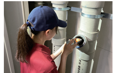
Testing water passage in pipes with testing tool
