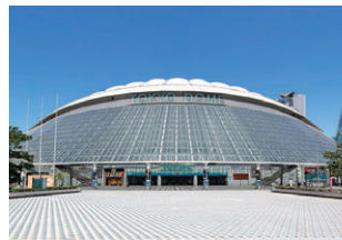
Tokyo Dome Air conditioning System
