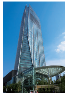
Toranomon Hills Mori Tower Air conditioning System
