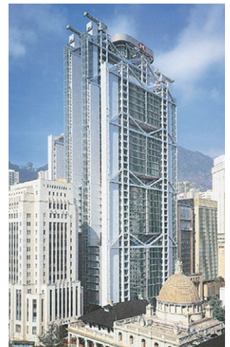
The Hong Kong and Shanghai Banking Corporation Limited, HSBC Main Building Air conditioning, sanitation and electric System (Hong Kong)
