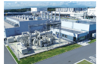
Kiyohara Smart Energy Center Civil Engineering and Construction of Plant Facilities
