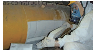
Removal of Piping Insulation Containing Asbestos
