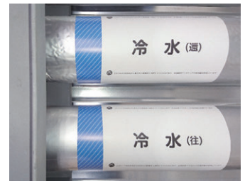
Image of piping identification sheets
