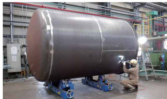
Welding work at Takahama Plant
