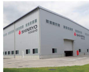
Exterior of Hiratsuka Plant No. 1
