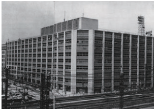
Shin-Otemachi Building Air conditioning System
