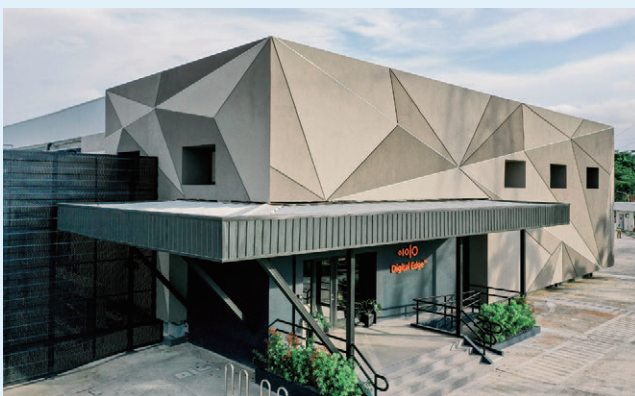
NARRA1 Data Center (Philippines)
