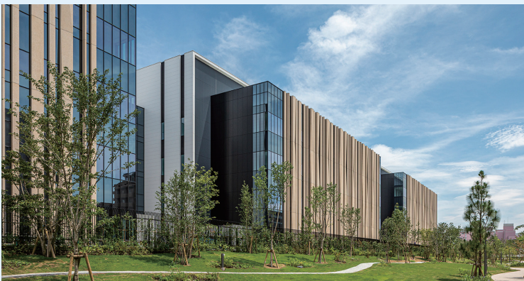
Chugai Life Science Park Yokohama (Yokohama City, Kanagawa Prefecture)
