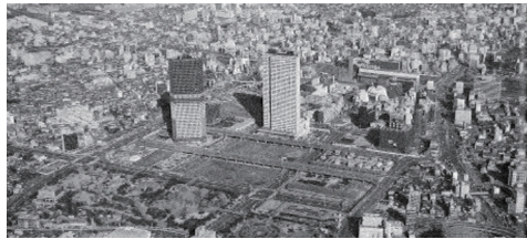
Shinjuku Fukutoshin District District Heating and Cooling System
