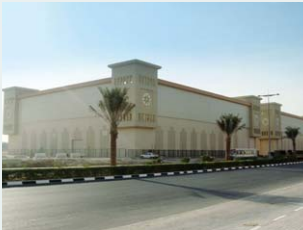
Discovery Garden DCS Plant (Dubai)
