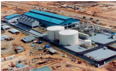
Kuala Lumpur International Airport CGS/DCS Plant (Malaysia) *CGS: Cogeneration System
