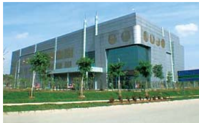
Putrajaya Precinct 1 DCS Plant (Malaysia)
