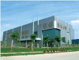
Putrajaya Precinct 1 DCS Plant (Malaysia)
