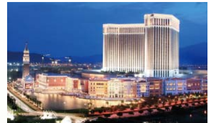
The Venetian Macao Resort Large Scale Chiller Plant (Macau)
