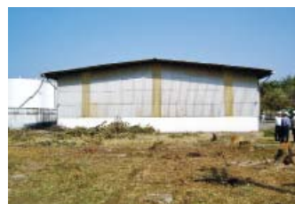
Warehouse before asbestos slate tile removal
