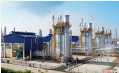
Petronas Penapisan (Melaka) Sdn Bhd Cogeneration Plant (Malaysia)
